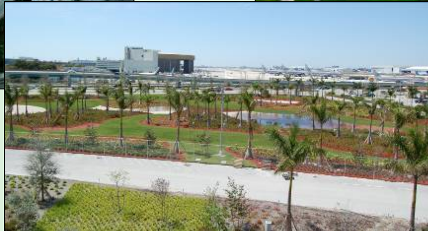
RCC Retention Pond →
